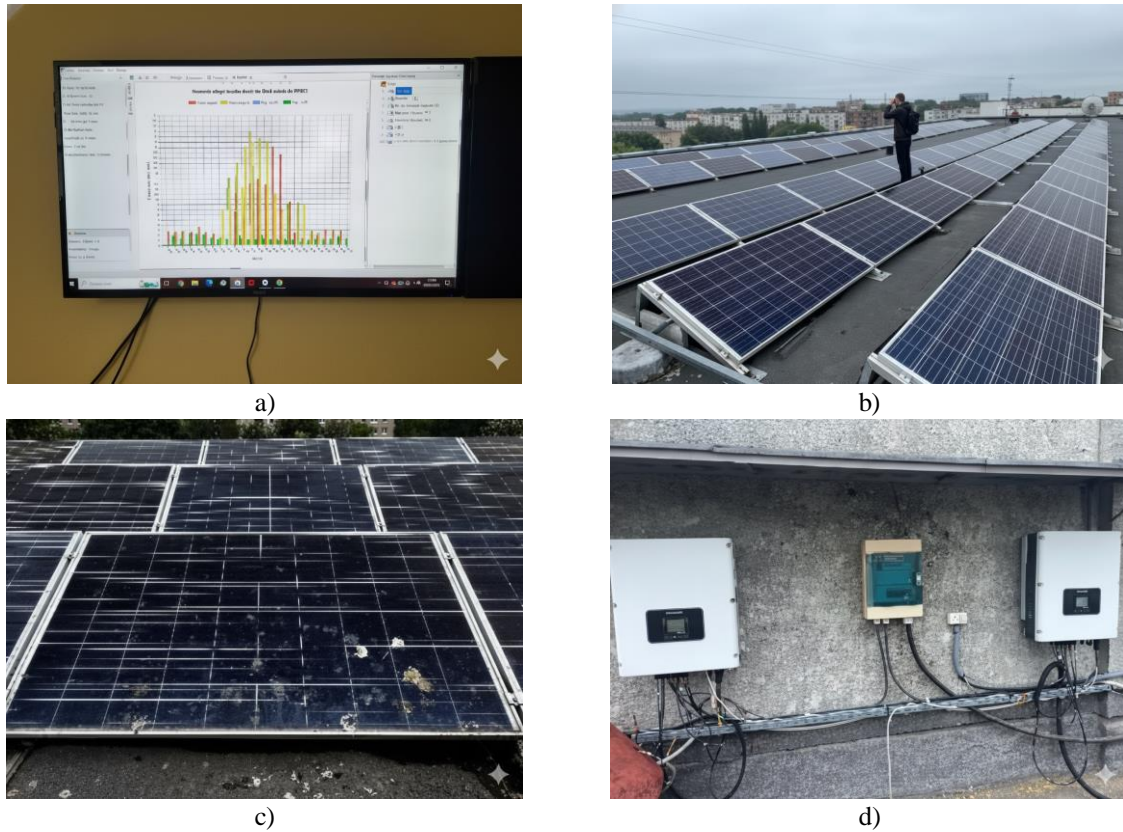
Fig. 8. Overview of the field validation setup: a) monitoring interface displaying real-time data from the survey; b) on-site manual inspection with portable thermal equipment for ground-truth verification; c) aerial view of the solar power plant under survey by the UAV; d) close-up of inverter and connection hardware being inspected
